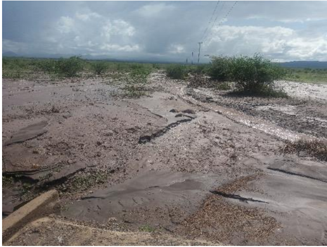
Figure 4: Silt carried by floodwater blocking drainage channels
