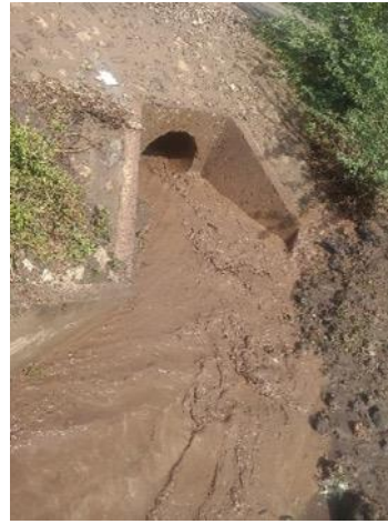
Figure 4: Silt carried by floodwater blocking drainage channels
