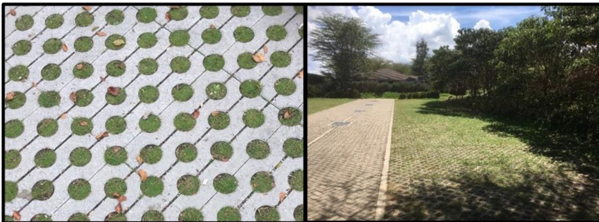
Figure 7: examples of permeable paving
