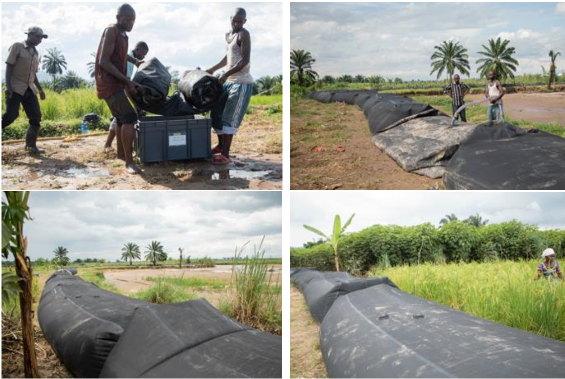
Figure 9: Example deployment of a water-filled barrier to prevent floods
